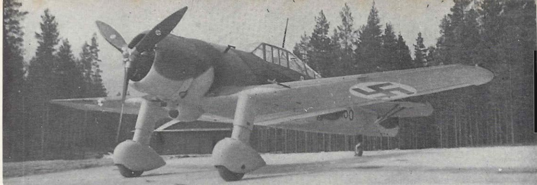
Above: The first V.L.-built Fokker D.XXI with Pratt and Whitney Twin Wasp Jr. engine and all-wing mounted armament. This aircraft has been finished in the black and green camouflage scheme, but carries no yellow identification markings, indicating that this photograph was taken before the start of the Continuation War. The aircraft is FR-150. (G. Kamphuis).
