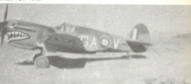
Below: AK772, a No. 112 'Shark' Squadron Kittyhawk Mk.Ia, showing the complete squadron markings. Note the serial has been left on a dark green patch; 'London Pride' in small white script above Y. Extended fuse on 250lb bomb, Gambut, 1942. (IWM)
