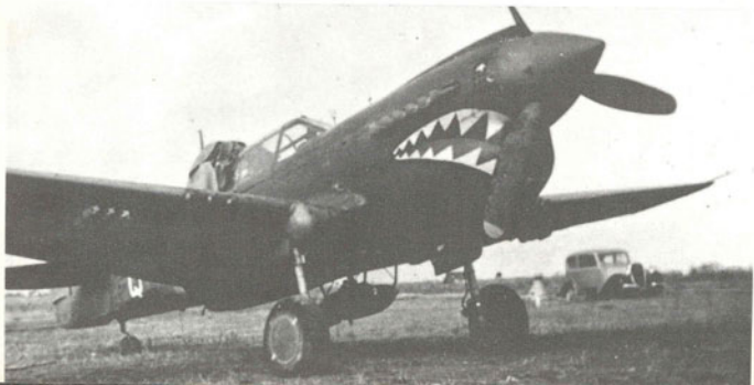
Below: One of the very few Kittyhawk Mk. IV's to be flown by No. 112 Squadron in USAAF OD and grey scheme. Red/black mouth, black lips, white teeth. Note 2 x 250lb bombs side by side under fuselage and 6 x 40lb under wings. GA-Q, FR806, Foggia Main, Italy. (via R. A. Brown)
