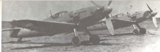
Left: S-199-(Bf.109G). A total of 422 were built by Avia during 1946-49 and 129 by Letov during 1948-49, all with the Junkers Jumo 211F engine.
