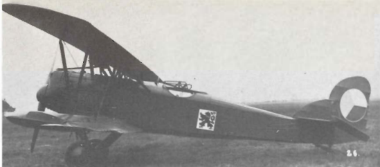
Letov S-6 bomber of 1923 powered by a Maybach Mb.IVa engine of 260h.p., 1st Air Regiment.
