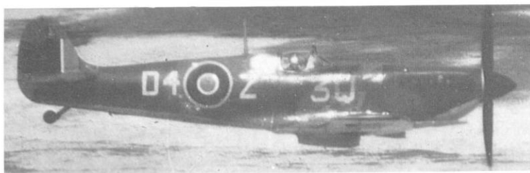
Seafire L.IIC, No. 809 Squadron, note two codes, 3Q— 808 Sqdn; D4— 809 Squadron. See colour illustration. (via R. C. Jones).
