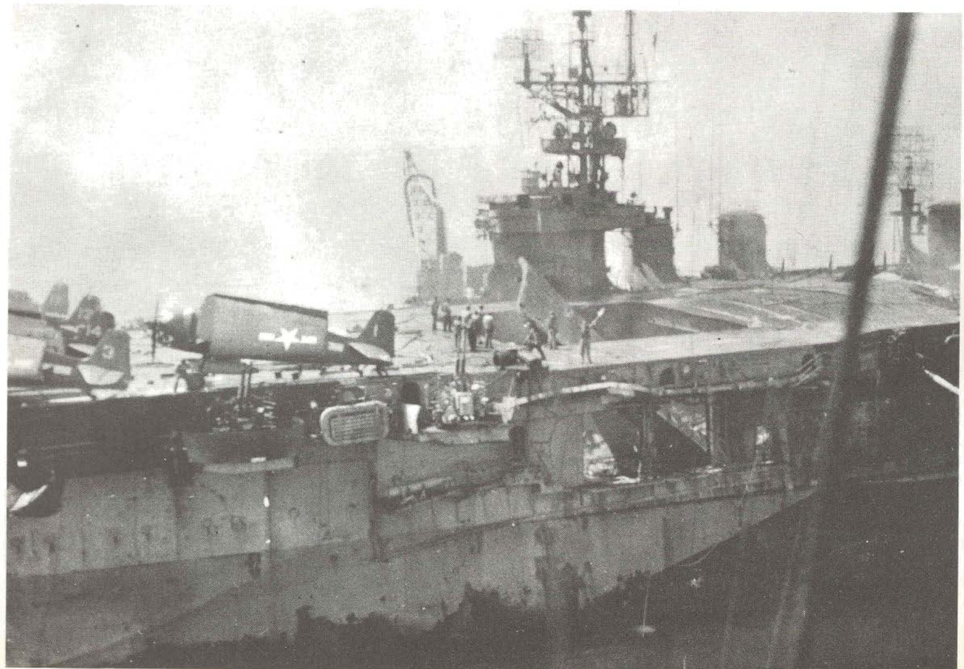
Below: A single bomb from a lone Judy resulted in this damage, and the sinking several hours later, on 'Princeton' in the "Battle of Leyte Gulf" on 24 October, 1944. The F6F-5, No. 1, on which the snarling face is just barely discernable, was that of CAG-27, Lt. Cdr. F. A. Bardshar. (US Navy)
