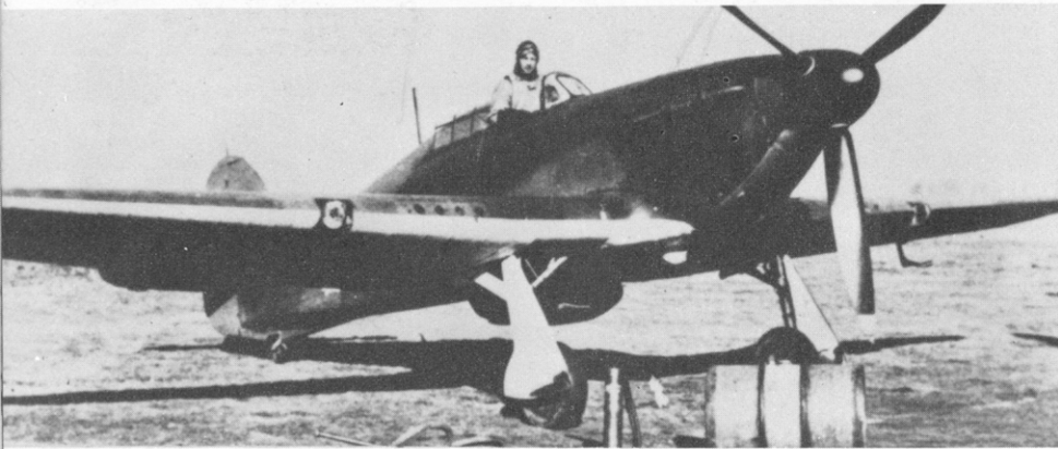
Belgian Hurricane Mk. I with Rotol propeller. (Lt.-Col. M. C. Terlinden)
