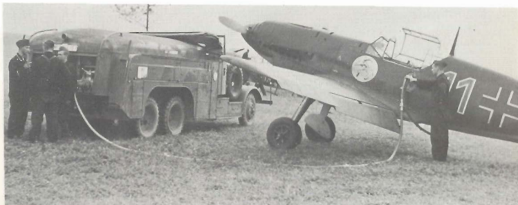
Above: Red 11 being refuelled, Bf 109B of JG 137.
