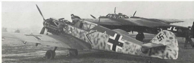
Below: The Gruppen-Adjutant's Bf 109E-3, II./JG 54, photographed alongside a Do 17Z in mid-1940. Note the red cross marking and stencilled numbers from 1 to 8 along the lower fuselage.
