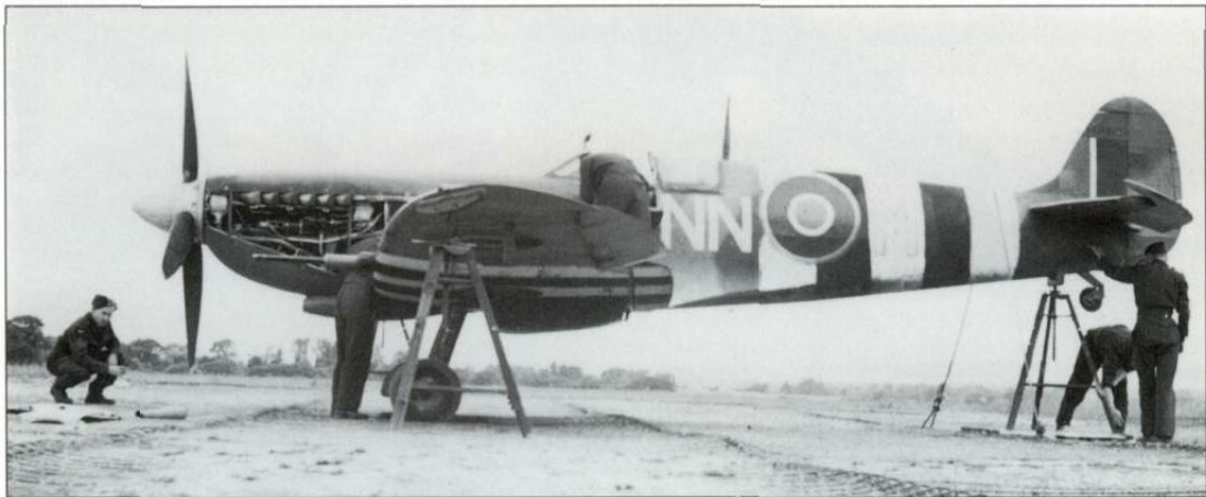
A Spitfire Mk IX of No 310 'Czech' Sqn is levelled off on a tail jack prior to the all-important harmonisation of the gunsight and guns taking place. A common occurrence on fighter stations across the UK during World War 2, this photograph was taken at Appledram, home for elements of the Tangmere Wing, in June 1944 (Hurt)
