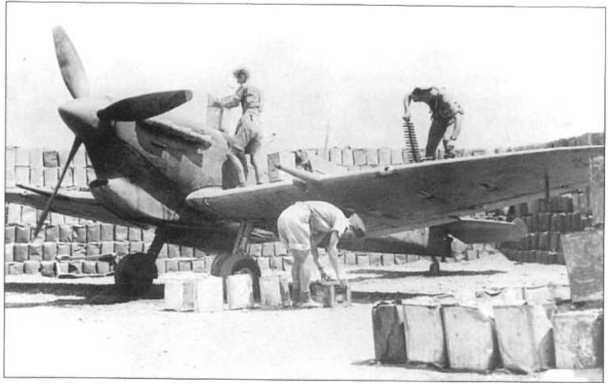
A soldier, a sailor and an airman carry out the refuelling and rearming of a Mk VC of No 603 Sqn in a makeshift revetment at Takali, Malta. Note that this aircraft has had the inner 20 mm cannon removed and the gun ports filled with locally made wooden bungs – its outer .303-in machine guns also appear to have been removed (via Robertson)
