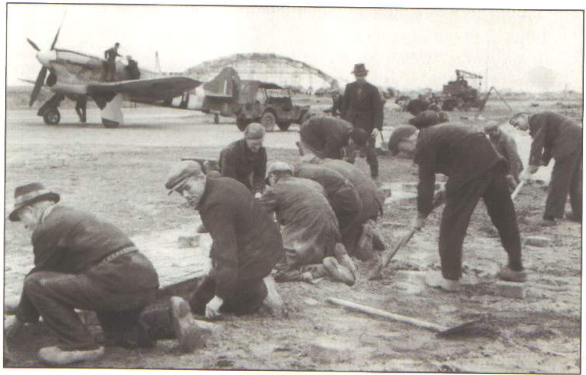
Much repair work on the damaged Dutch airfields was undertaken by local labour, who laid thousands of bricks to form taxiways, dispersals and even runways. In the background a Tempest (believed to be 'H' of No 3 Sqn, EJ or JN817) receives attention (IWM CL1415)
