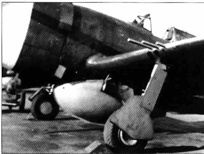
The use of external fuel tanks greatly increased the effective bomber escort range for VIII Fighter Command P-47s. The 'bathtub' ferrying tank – seen here fitted to a 335th FS/4th FG Thunderbolt – was the first type of external fuel source employed in the ETO. Proving prone to leakage and sometimes failing to release in flight, the 'bathtub' tank (nicknamed the 'baby' by pilots) was only used for a handful of missions in August 1943 (via Dick Martin)
