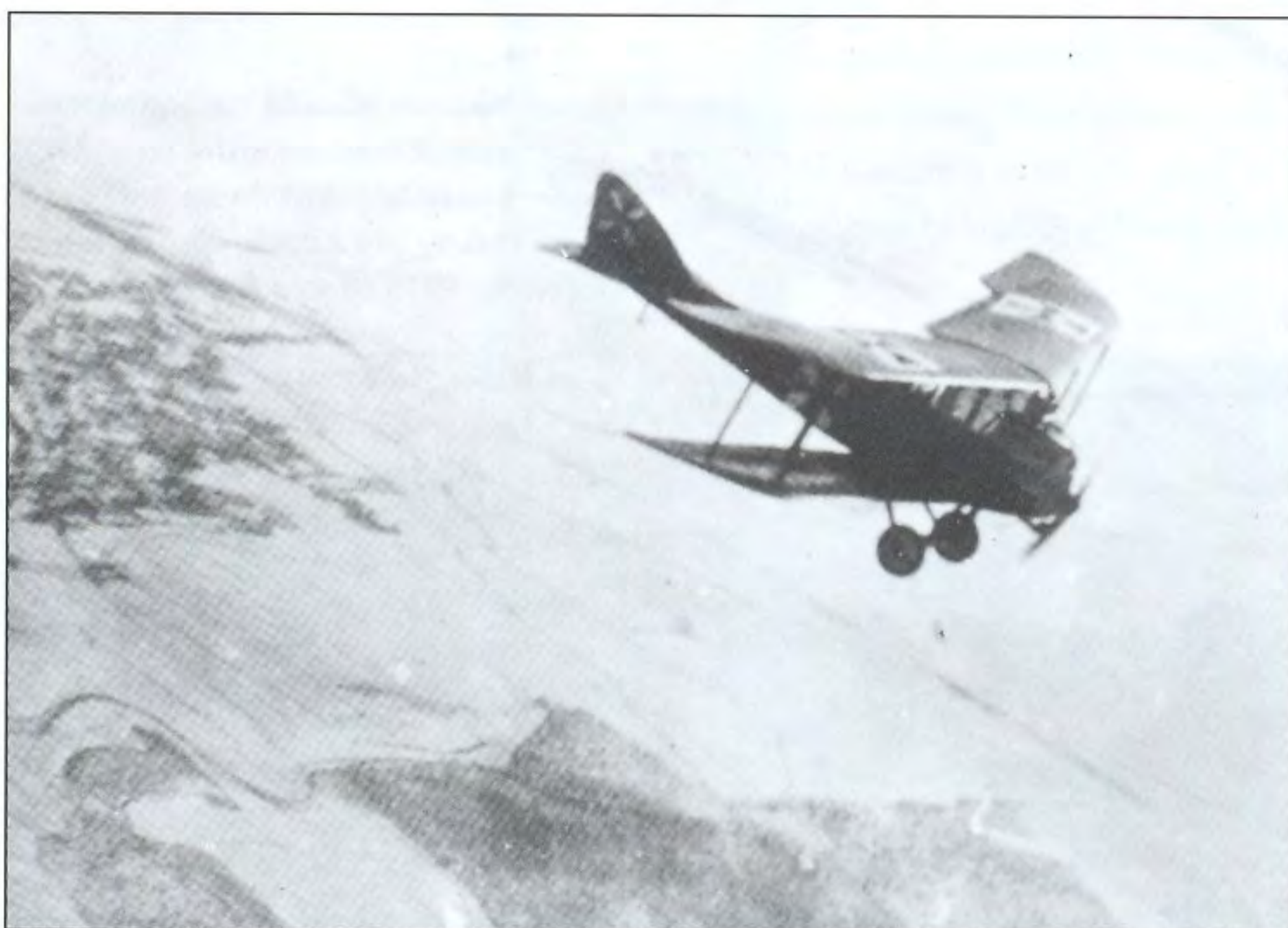
This rare air-to-air photograph of air activity over the Eastern Front depicts one of the 24 Oeffag C I two-seaters that were built as the 51 series with a 112 kW (150 hp) engine before the advent of the C II (52 and 52.5 series) with 119 or 134 kW (160 or 185 hp) engines respectively (Bruce Robertson)
