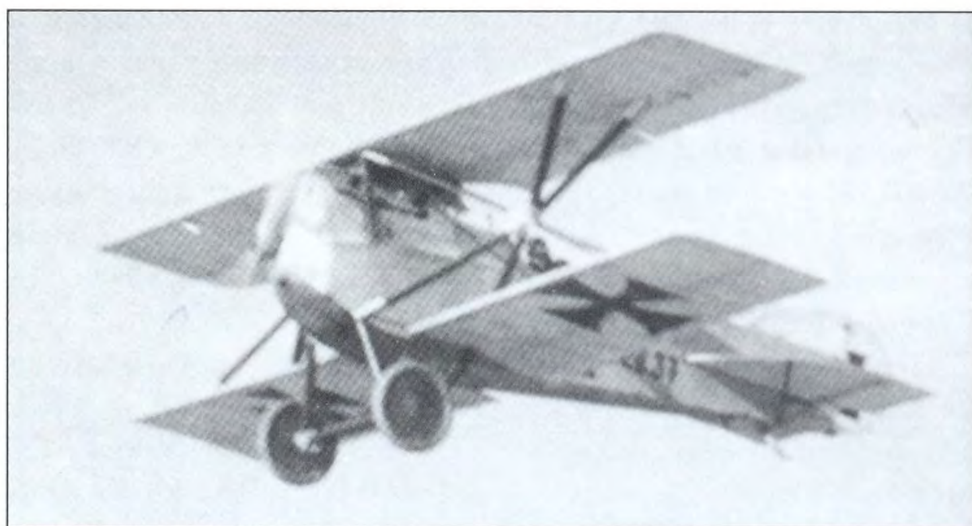
This Hansa-Brandenburg D I (28.37), flown by Kiss, was one of the few examples of this 'star-strutter' fighter fitted with a synchronised Schwarzlose machine gun in the upper part of the forward fuselage rather than the original armament of one unsynchronised machine gun in a fairing above the upper-wing centre section. Another feature of this aeroplane was the low-aspect-ratio fixed fin added to the upper fuselage ahead of the rudder for improved directional control (Bruce Robertson)
