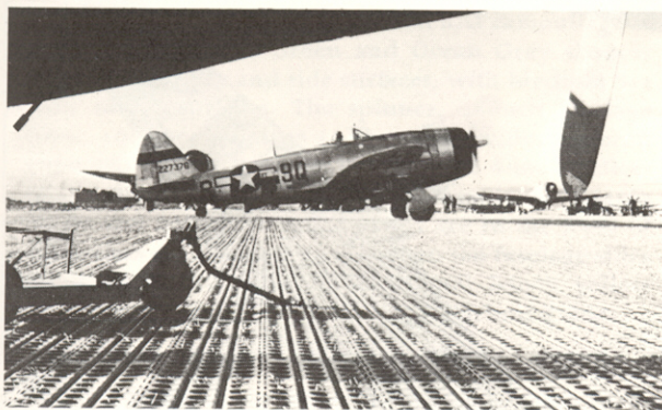
27. The use of pierced-steel planking enabled Engineer Aviation Battalions to build advanced air bases in less than two weeks. One of these bases is seen used by P-47D-27-RAs of the 404th Fighter Squadron, 371st FG, First Tactical Air Force (Provisional). (USAF)
