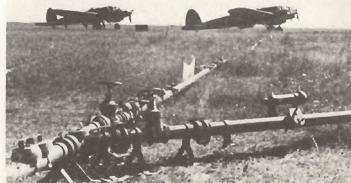
53. Complex fuel lines such as these were necessary on the Eastern Front, where airfield facilities were often limited.
