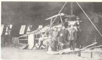
S.E.5a F5611 undergoing extensive repairs, including an engine change in No. 56 Sqn.'s workshops. Note the tripod for hoisting engine clear of mounting. (J. Cooper)
