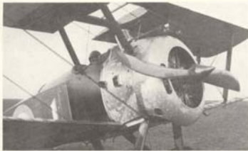
Sopwith Camel of No. 210 Sqn. A 150hp B.R.1 rotary-engined aircraft, it has the white fuselage number '1' with a blue shadow. (R. Sykes)
