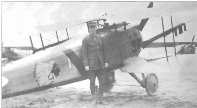
Adjutant Walter Lovell beside his SPAD VII, which is evidently undergoing maintenance – note exhaust stacks resting on the flying wires (Lafayette Foundation)
