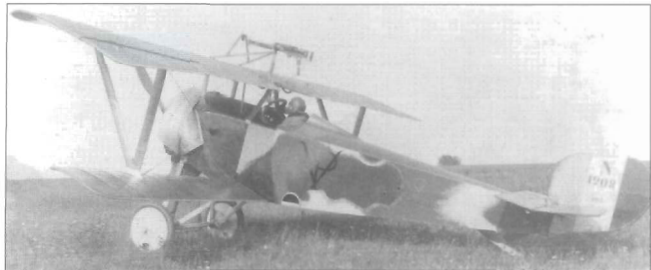
Sgt Paul Pavelka's Nieuport 11 N1208 displays an unusual, non-standard camouflage pattern and monogram emblem, probably in red (National Archives)
