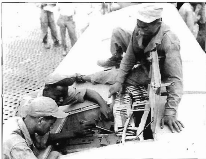
Armourers re-arm one of the group's P-51B/Cs (a hand-me-down from the 52nd FG, judging by its wing bands). The angled installation of the P-51B/C's guns led to jams – something the 332nd's armourers had to contend with until VE-Day ( National Museum of the USAF )
