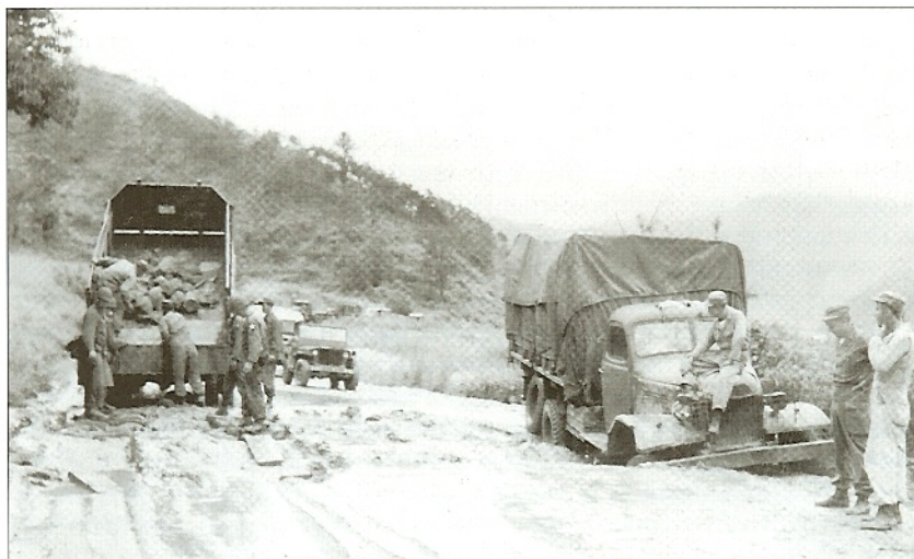
Road transportation in Korea was a challenge. Rains washed out this road, part of the main supply route (MSR), July 27, 1952. 2d Infantry Division Engineers make a temporary repair. (MHI)
