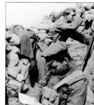
The Expeditionary Force fought over ground with a very high water table, which meant that any hole dug too deeply would quickly fill with water. To avoid this, many ‘trenches’ were not trenches at all, but earthworks made of sandbags. (Imperial War Museum, Q49369)
