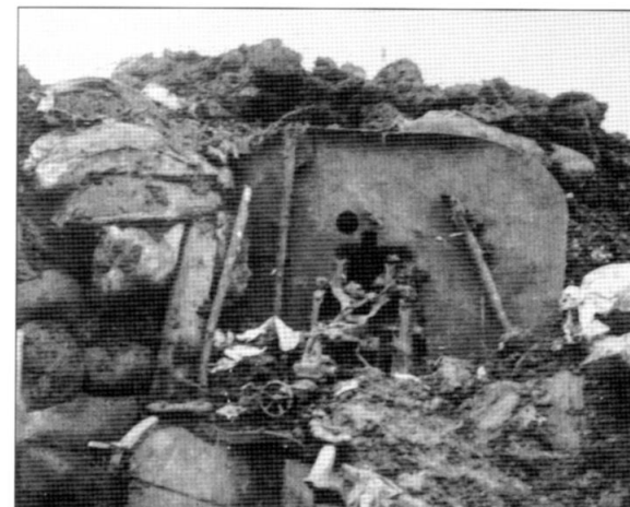
This German machine-gun position was destroyed by a British howitzer shell that fell on top of it during the battle of Neuve Chapelle. Had the position been hit by a shell fired by a field gun, the sandbags in front of the position would have been damaged, but the position itself would have remained intact. (Imperial War Museum, Q49208)
