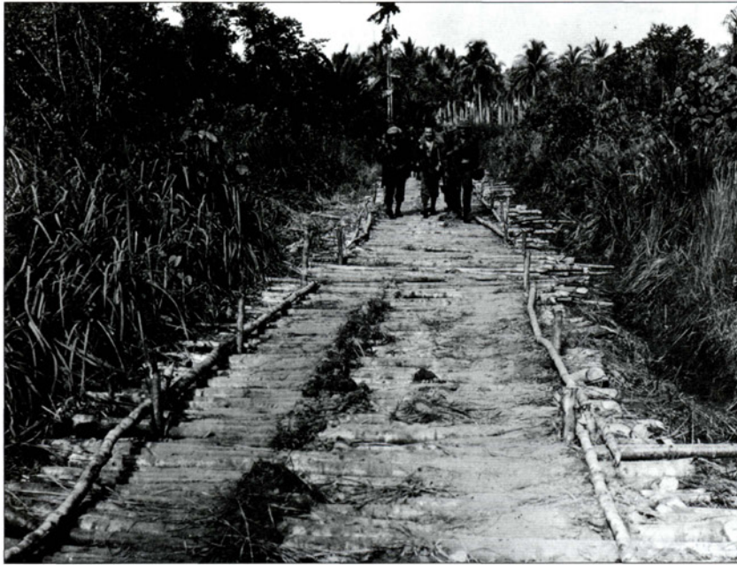
A corduroy road built by the 114th Engineer Battalion, 32d Division to allow jeeps to carry supplies and ammunition over swampy areas, December 21, 1942. This road runs from Dobudura to Buna Village, New Guinea.
