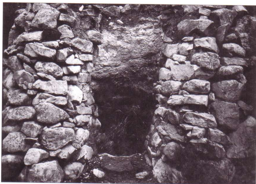
Once the Republicans were established in the hills around Auts, defences were built in order to defend the area. This position is one of a number in the area which survive and are built from stone with a deep well to protect the occupants from shrapnel or small arms fire. (Author's photograph)
