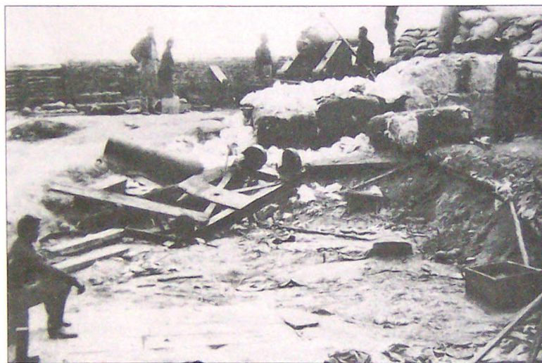
ABOVE The High Bastion marked the northeastern corner of the Confederate defenses around Yorktown. Built on top of a British redoubt dating from the Revolutionary War, this bastion could enfilade an enemy assaulting the main defensive line. In this photograph, taken in May 1862, the viewpoint is from the top of the river bluff, to the northeast of the Confederate position.
