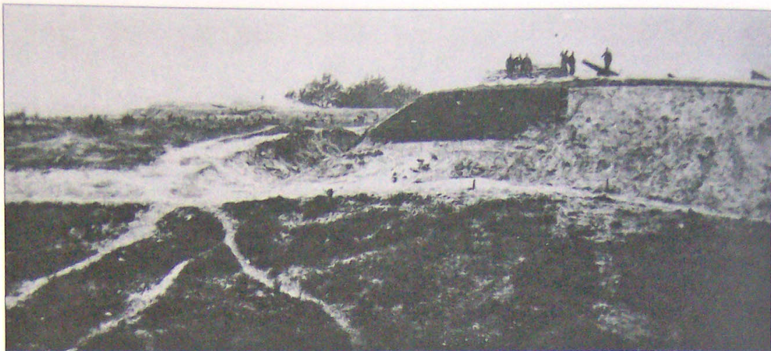
ABOVE The High Bastion marked the northeastern corner of the Confederate defenses around Yorktown. Built on top of a British redoubt dating from the Revolutionary War, this bastion could enfilade an enemy assaulting the main defensive line. In this photograph, taken in May 1862, the viewpoint is from the top of the river bluff, to the northeast of the Confederate position.
