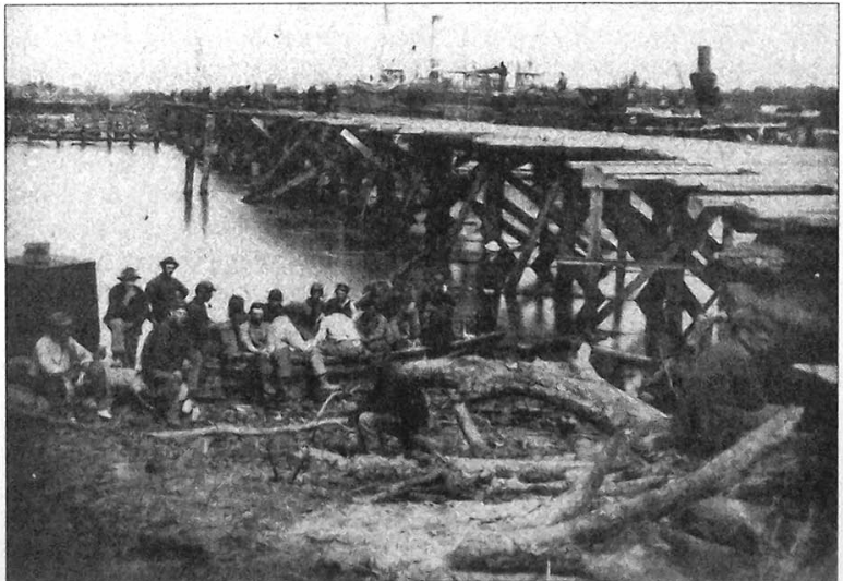
The Railroad Bridge over the Pamunkey River was quickly repaired by Union engineers, and the Richmond & York River Railroad was pressed into service to haul Union supplies to the army encamped astride the Chickahominy River. Note the railroad engine on a barge in the background; another example of the phenomenal logistical resources available to McClellan. (National Archives)
