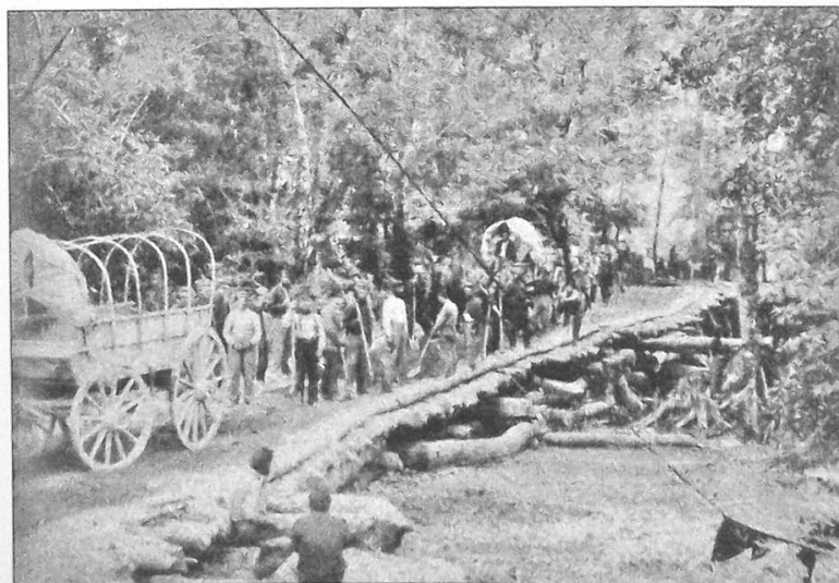
The Army of the Potomac had to commit considerable effort and resources to the supply of its soldiers in the Tidewater Peninsula. In this view of the approach to Grapevine Bridge over the Chickahominy River, a "corduroy" road of felled logs has been laid over a raised trestle approach road to the river. (Library of Congress)
