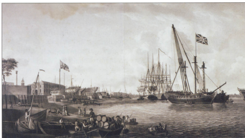
Deptford shipyard on the Thames. One of several facilities run by the Navy Board, such yards constituted the largest industrial enterprises of their day anywhere in the world. Deptford had five slips for the construction of warships and was capable of building at least one first rate at a time. (Royal Naval Museum, Portsmouth)
