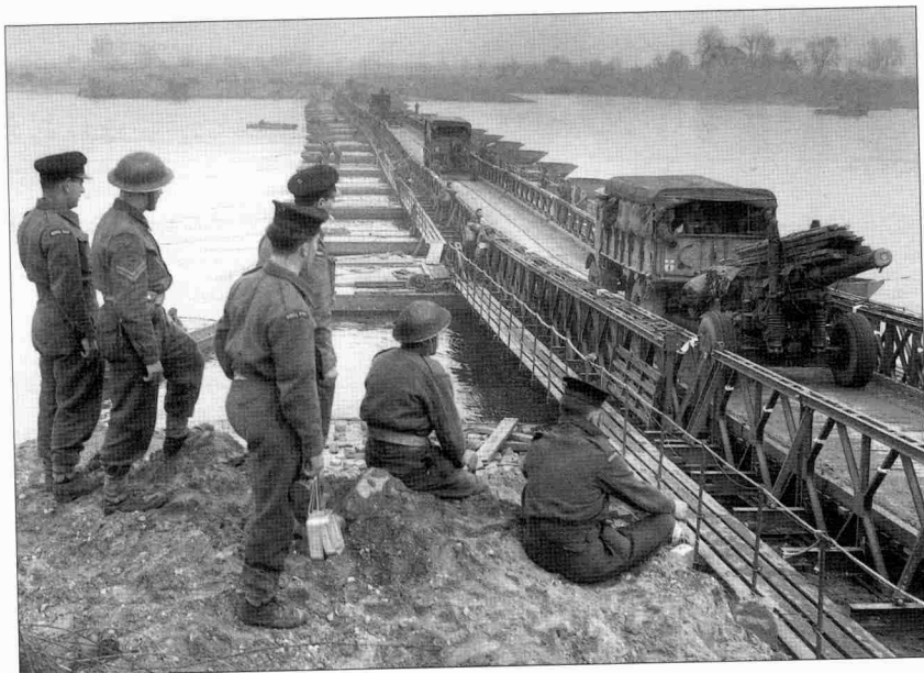
Guns from one of Second Army's medium artillery regiments cross over the Rhine on a newly completed Bailey bridge. (BU 2392, IWM)
