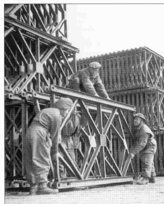
Bridging operations on the River Rhine were the most complex of the war. Great stockpiles of Bailey bridging material were assembled prior to the attack. (B 15755, IWM)
