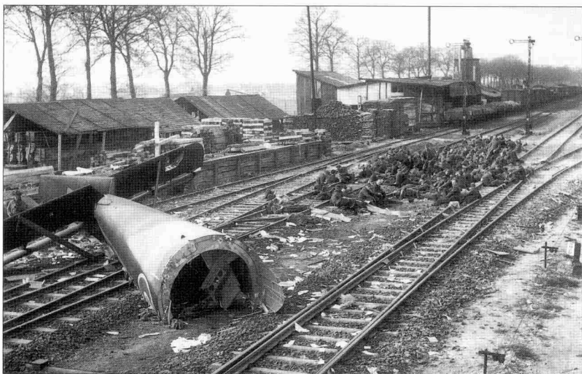
The rear end of a British Horsa glider straddles the railway line near Hamminkeln railway station. In the background a party of German prisoners wait to be moved to the rear. (BU 2305, IWM)
