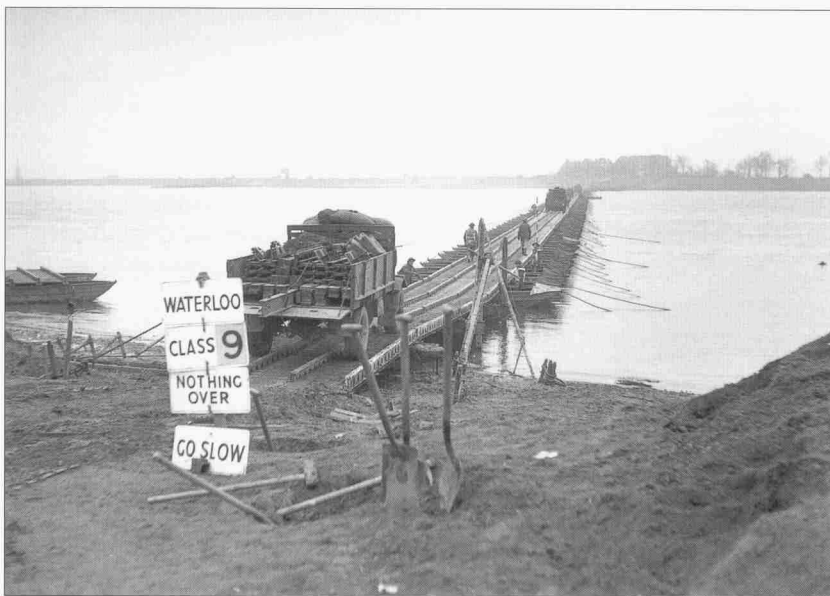
British transport crosses XXX Corps' 'Waterloo' Class 9 folding boat bridge, built downstream of Rees by 18 GHQ Troop's Royal Engineers. It was open to traffic at 0200hrs on 26 March. The bridge classification means that only loads of up to 9 tons are able to use the bridge. (BU 2717, IWM)
