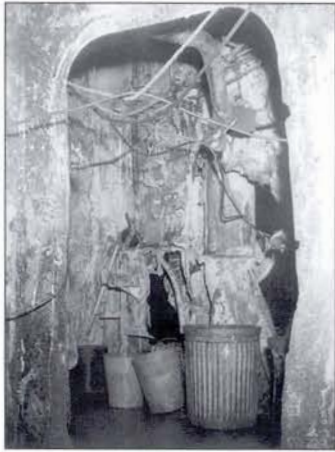
Where it started – the flare locker shows the blowtorch effect of the inferno
