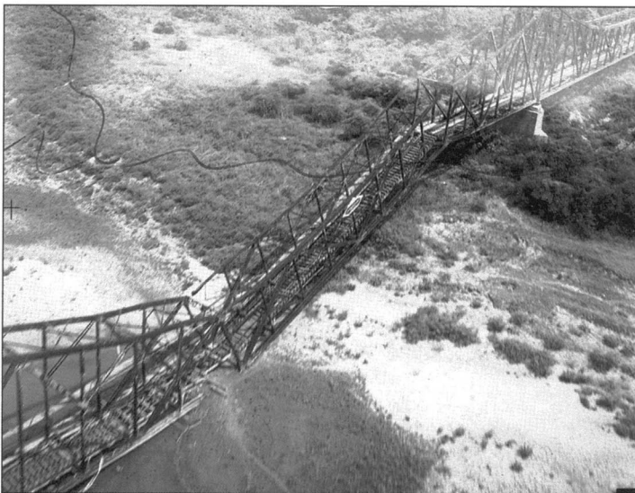
A bridge on the central Siam railway, near Uttardit, was destroyed by aerial bombardment, and photographed on 29 March 1945 from 100 ft (Stevens Collection)
