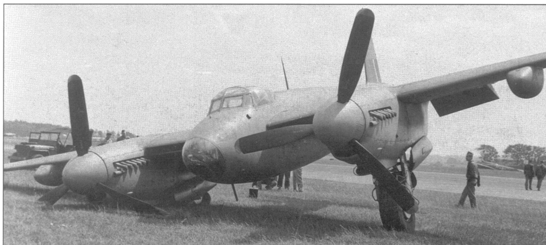
'Just dropped in old boy!' PR XVI NS553 suffered a starboard undercarriage failure after putting down in an emergency during the summer of 1943 at the 96th BG base at Snetterton Heath, in Norfolk (via Dick Jeeves)
