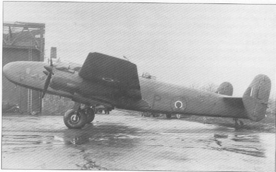
The same aircraft is seen later in its career, with extended inboard engine nacelles and a modified, streamlined nose (Author's collection)
