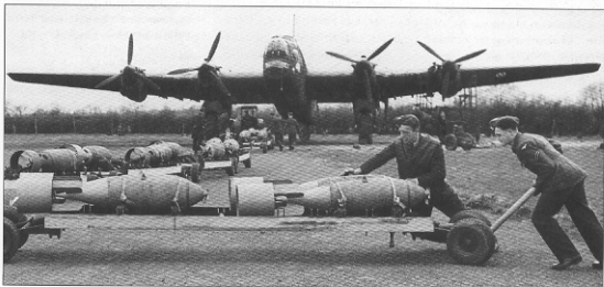
Armourers struggle with a bomb trolley – one of six waiting for loading of the 24 500-lb bombs aboard this Merlin XX-engined Halifax. Special, purpose-designed, target markers were soon developed for use by the Pathfinders, who also dropped incendiaries, and even continued to use some HE bombs like these (via Phil Jarrett)
