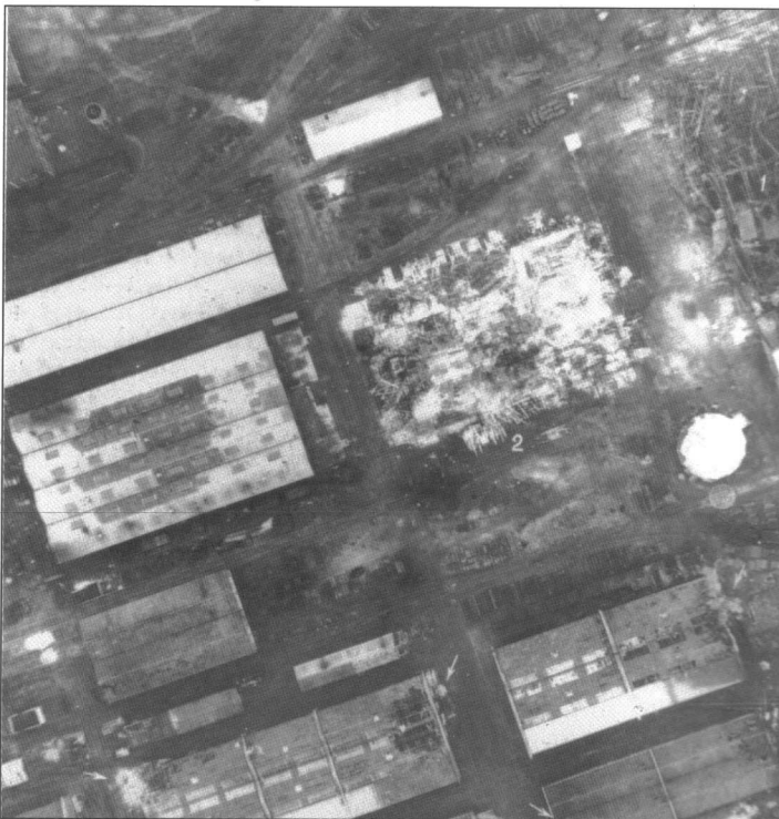
This reconnaissance photograph shows further damage at Le Creusot, where many buildings were destroyed by direct hits. These are the processing works and locomotive machine shop (via Francis K Mason)
