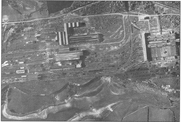
A post-strike photograph showing extensive damage to the Breuil Steelworks at Le Creusot. The general machine shops (bottom) were straddled by a stick of 1000-lb bombs, the steel manufacturing plant and sheet and bar mills badly hit and a 650-ft warehouse entirely destroyed (via Bruce Robertson)
