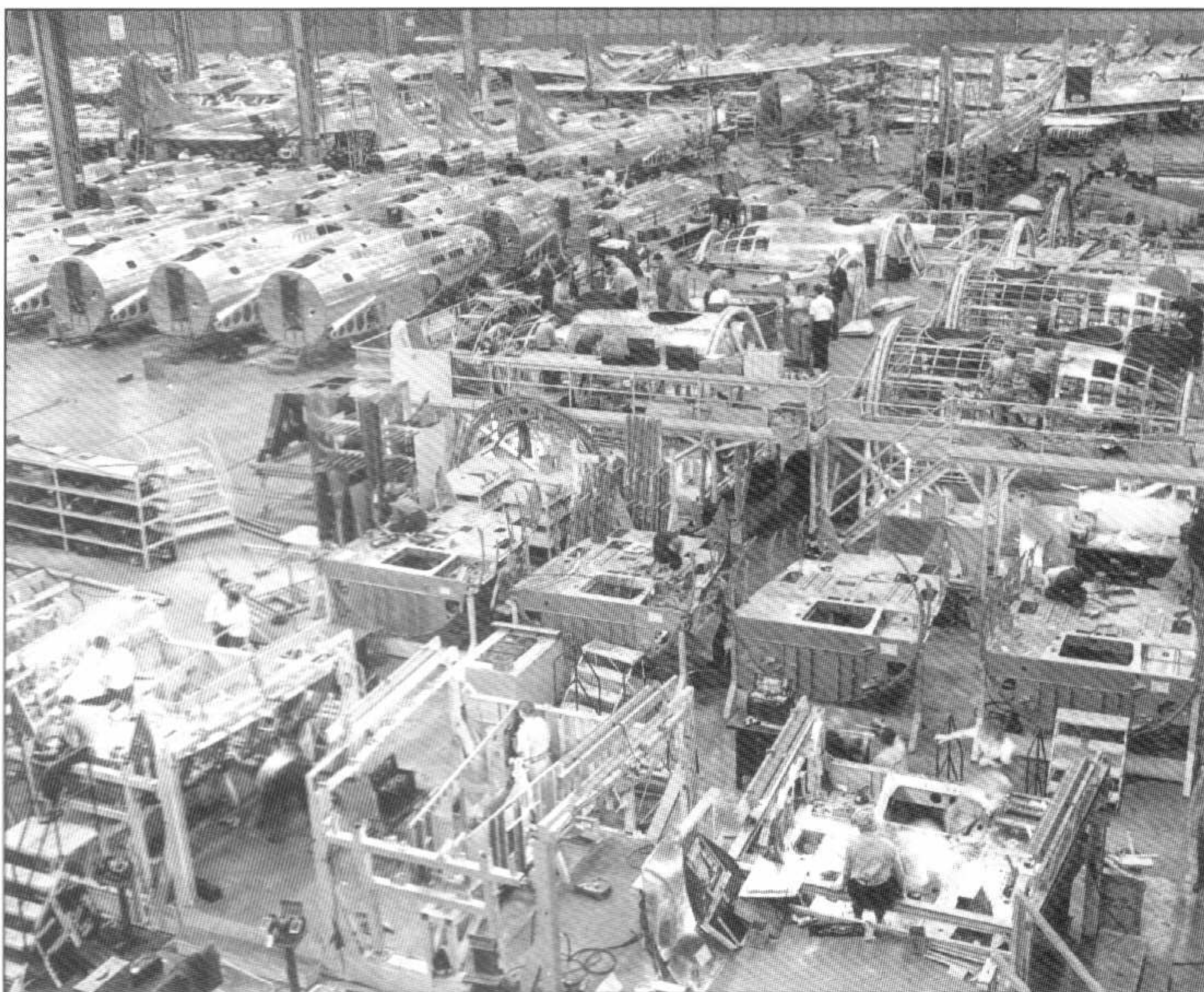
The Boeing plant at Renton is seen during its changeover phase from the B-17 Flying Fortress to the B-29 Superfortress. Construction of the B-17 is continuing in the background, literally surrounding jigs for the B-29 in the foreground. (Boeing)
