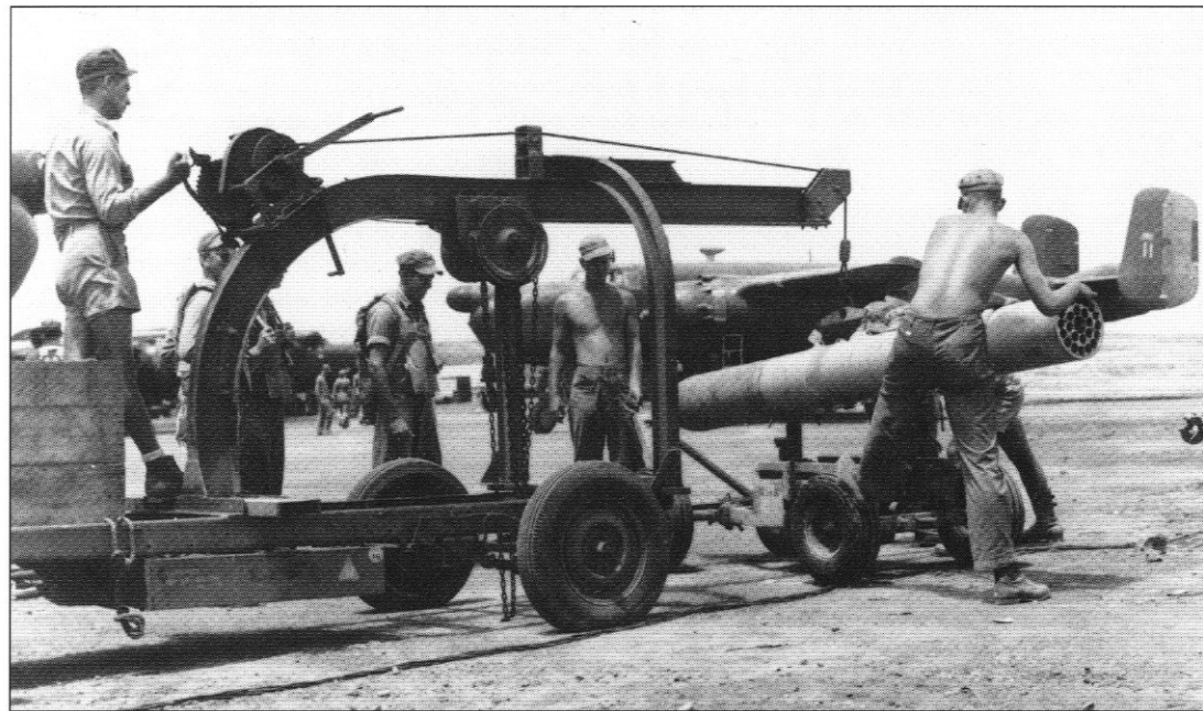
A modified truck hoist is used to swing the rocket onto its special wheeled trailer (National Archives)
