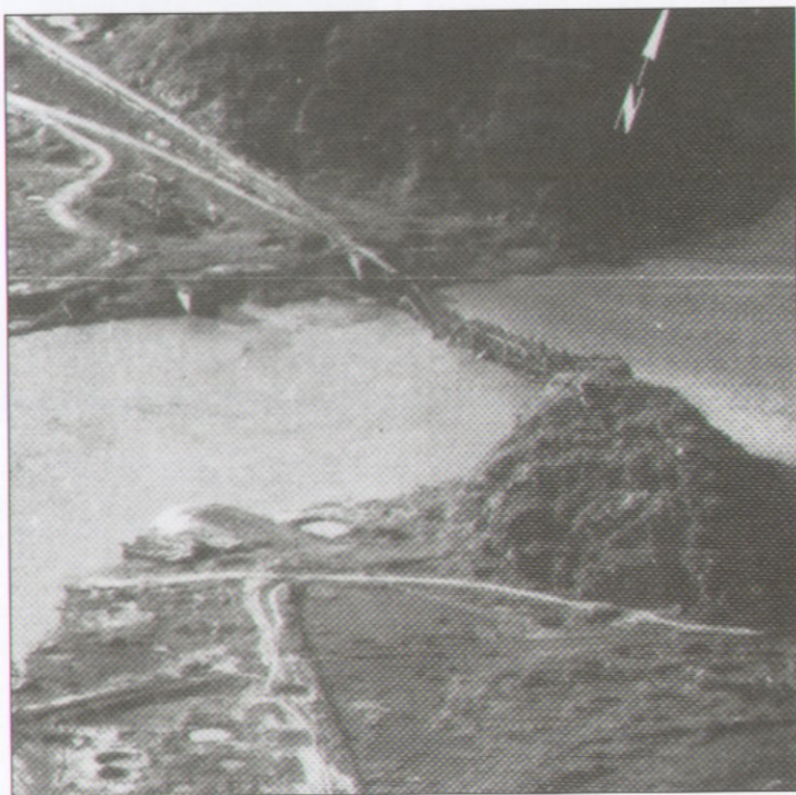
Post-strike photography shows the fabled Thanh Hoa span down
