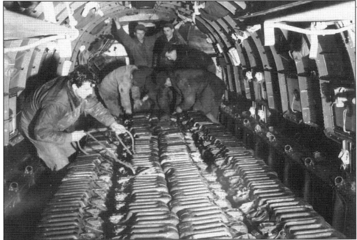
An internal view of a C-47 loaded with five-gallon jerrycans bound for an airfield at Orleans, in France, in the late summer of 1944. Although not an efficient or safe way of lifting gasoline – filling and static discharge accidents claimed a number of C-47s – the fuel airlift was critical to the Allied advance across France in the summer of 1944 (National Archives)
