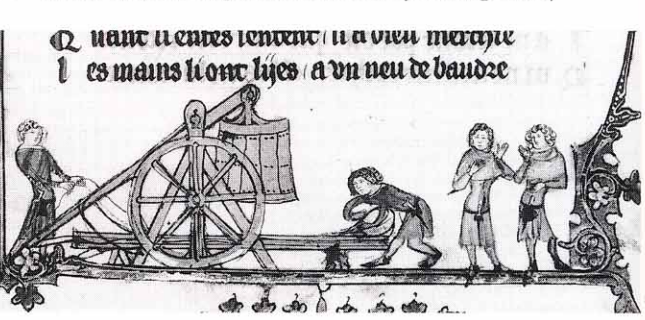
(1) A ballista or giant catapult, from the manuscript of Walter de Milemete dated 1326. The powerful bow is tensioned by the windlass at right. The wheeled ballista (2) is from the 'Romance of Alexander' of c.1330, and is bent by a screw. Here the arms appear to be separate and may have been held taught by skeins of twisted rope as used in Greek and Roman versions as shown in the 11th-century Byzantine drawing (3). The 16th-century illustration by Lipsius (4) gives a better idea of the appearance of the latter machine. (Oxford, Christ Church Ms.92, f.68v and Bodley Ms.264 f.201r)
