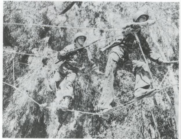
Marine raiders cross a bridge constructed of linked toggle ropes, a technique borrowed from the British Commandos. Carried by each raider, these consisted of an 8 ft.
