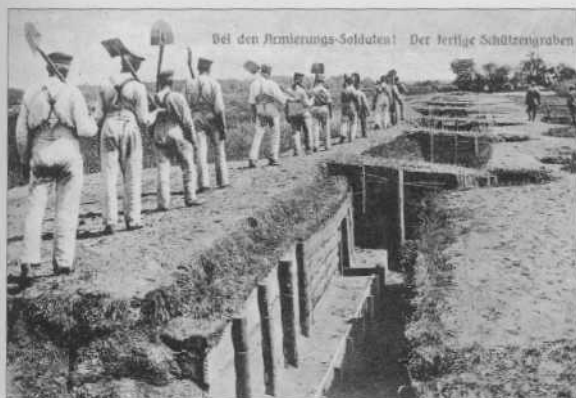
Pristine Schutzengraben – German fire trenches – dug by soldiers wearing white fatigue uniform. Note the timber revetment, fire steps, and traverses designed to limit the effects of blast and enfilade fire.
