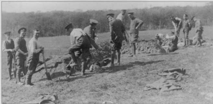
British troops demonstrate the ideal trench-digging method, with traverses marked out with pegs, and sods laid to cover the parapet.
