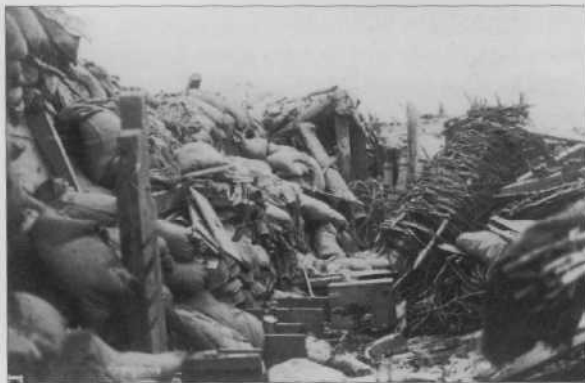
Trench smashed by shellfire, Argonne front - probably in the French lines. Wicker gabions have been torn up and the sandbagged walls have collapsed.
