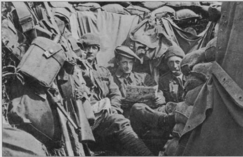
Men of the King's Own (Royal Lancaster Regt) make themselves comfortable; groundsheets and webbing festoon the trench walls, and note the parapet built up with courses of sandbags laid in alternate layers 'side-on' and 'end-on'. The men's headgear includes rolled-up balaclavas, and the 1914 'winter' unstiffened service dress cap with its distinctive flaps - the famous 'Gor-blimey'. (King's Own Collection, Lancaster City Museum)
