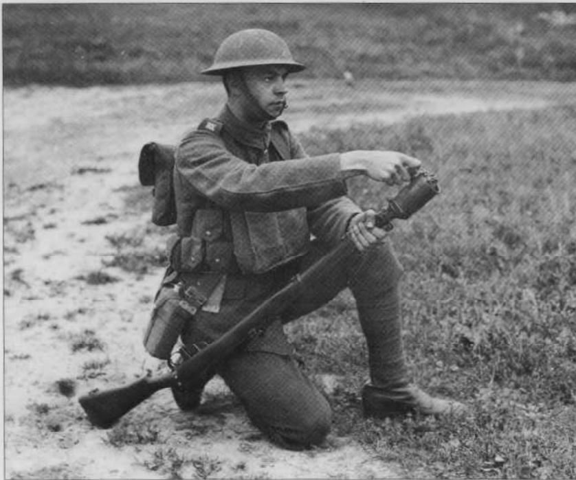
A Royal Engineer demonstrates the use of the No.36 Mills grenade with the cup discharger, 1917. With a range of 240 yards, the discharger was eventually issued on a scale of 96 per battalion. The rifle is held butt to the ground and trigger guard upward, and the grenade inserted into the cup so that the firing lever is confined after the safety pin is removed. It is discharged by firing a bulletless ballistite cartridge.
