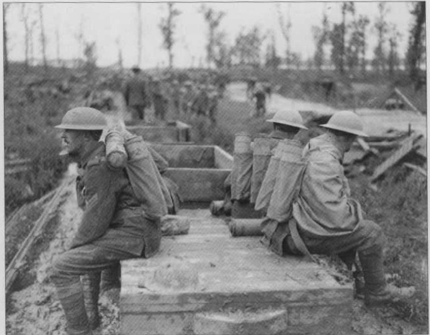
Ammunition carriers hitch a ride on a light railway from a shell dump to battery positions behind the front line. Nearly 1,000 miles of track were laid behind the British front during the preparations for major offensives, with more than 520 locomotives and 20,000 wagons under War Department control. (IWM Q5853)
