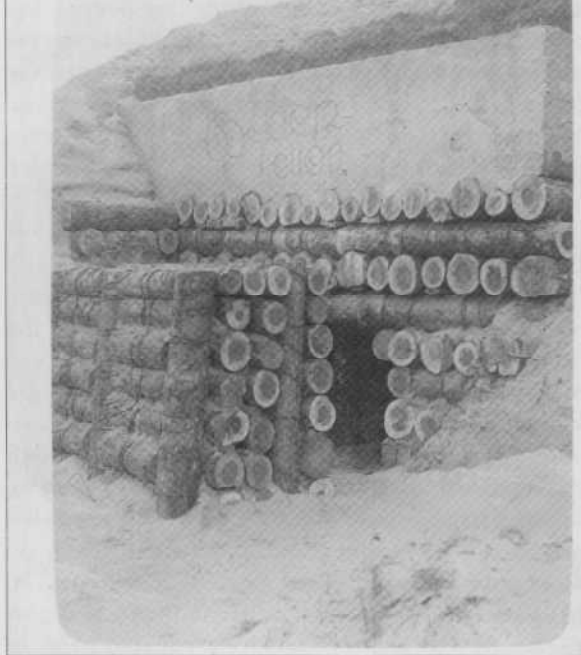
June 1917: an excellent view of the log and concrete Heiden-keller ('heroes' bunker) built at Hill 151 for the HQ of I Bataillon, Infanterie-Regiment Nr.422.
