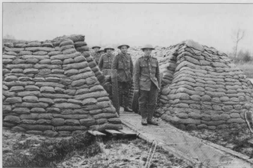
'Plugstreet' Wood, January 1917: men of the Lancashire Fusiliers emerge from a built-up section of 'box trench' onto a duckboard path. This is the rear entrance of a communication trench; in the coastal sector of Flanders, where the water table was very high, fire trenches also had to be constructed above ground in this way.
