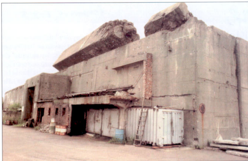
The exterior of the Elbe II bunker. The interior walls were blown out and the roof collapsed: its massive sloping slabs are clearly visible leaning against the top of the remaining wall.
