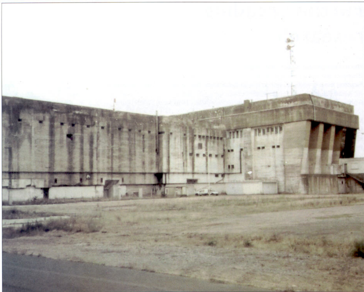
ABOVE The rear of the St Nazaire bunker today. The stains of nearly 60 years' exposure to the elements are the only signs of deterioration on this imposing edifice. (Chris Boonzaier)
