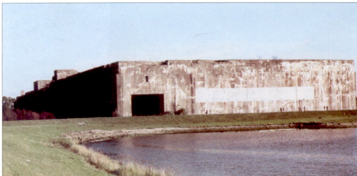
ABOVE The western face of the Valentin bunker. On the left is the entrance through which component sub-assemblies could be brought by barge and through which the completed Type XXI would exit into the River Weser. Since the end of the war, the
