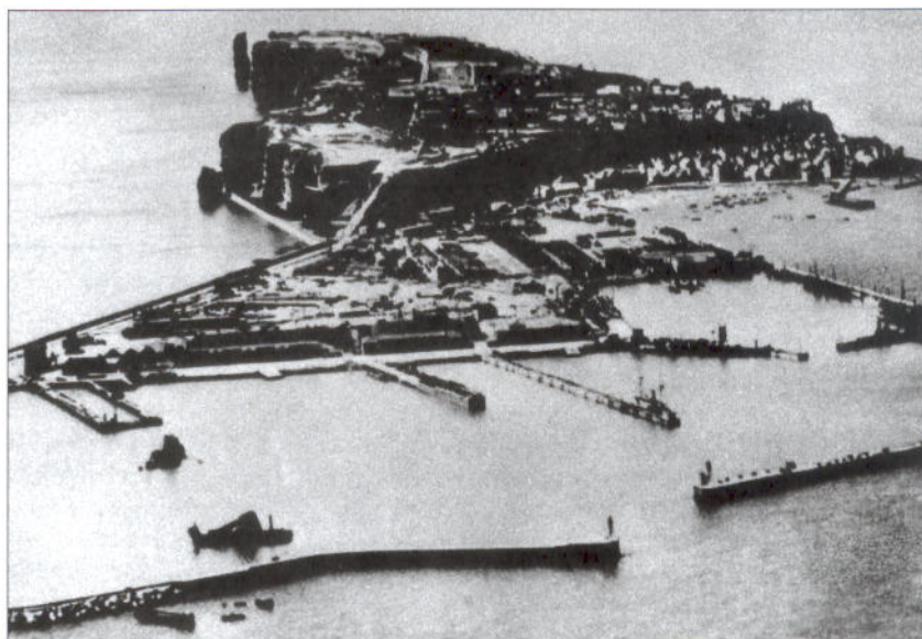
The island of Helgoland, site of numerous defensive structures, including a modestly sized U-Boat bunker.
