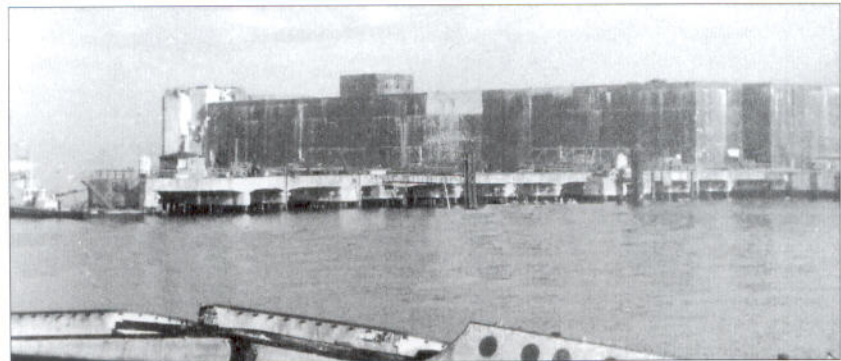
The Kilian bunker at the end of the war, just before its demolition by troops from the Royal Engineers.
