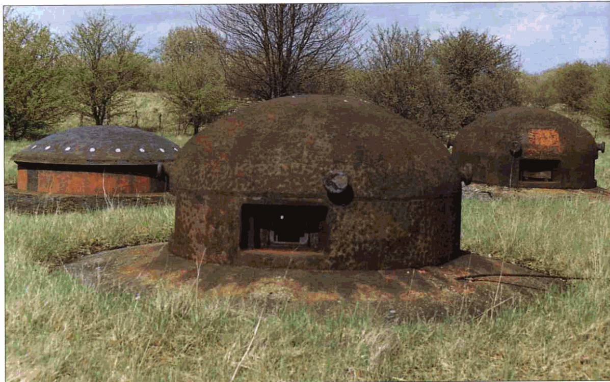
The surface of combat block 3 of the gros ouvrage of Rochonvillers. In the foreground and to the right can be seen the block's two armoured observation and automatic rifle cloches that provided part of the close-in defence of the ouvrage's surface. To the left is the block's artillery turret in the raised, firing position. It is armed with two M1932-R 75mm howitzers. (T. McGovern Collection)
