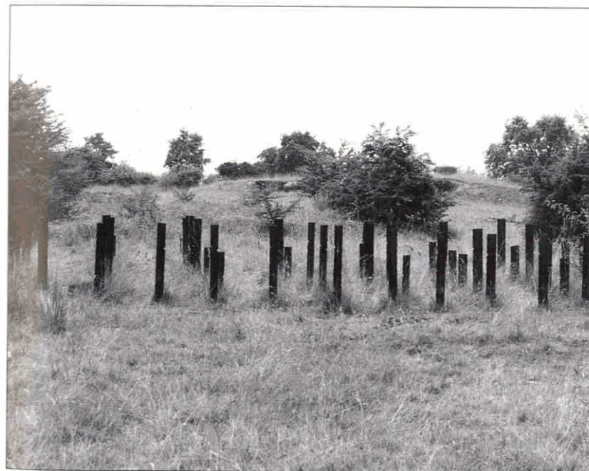
A section of the anti-tank obstacles surrounding the combat block area of the gras ouvrage of Four à Chaux. It consists of lengths of old railway rails set in concrete. Most other areas of anti-tank rails have long since disappeared. Two of the ouvrage's cloches are visible in the background. (Author's photograph)
