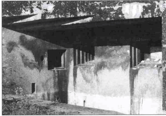
ABOVE LEFT The two primary firing embrasures of the interval casemate of Grand Lot. To the left is the smaller embrasure for an automatic rifle protecting the casemate's ditch. The weapons have been removed and embrasures have been boarded up. (Author's photograph)
