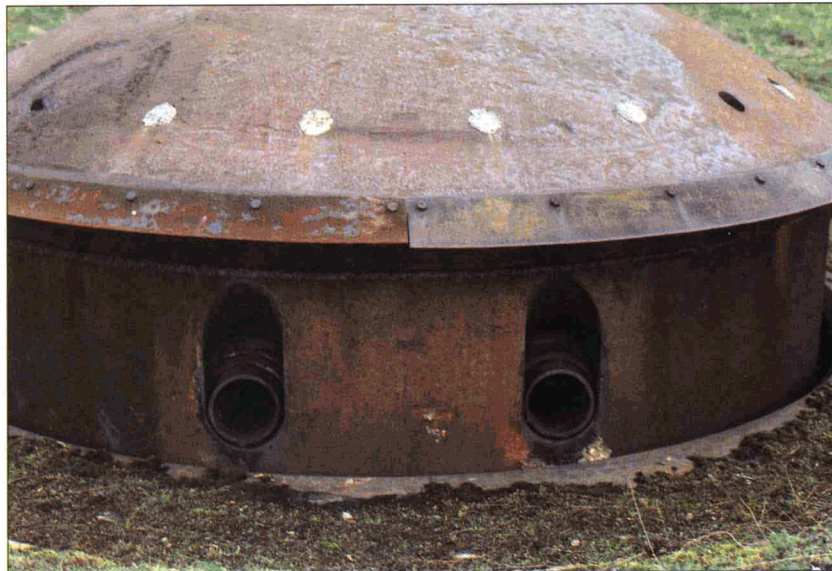
The business end of the 135mm howitzer turret of block 7 of the gros ouvrage of Rochonvillers. Note that there are no apertures for sights. All 135mm howitzer turret fire was indirect using elevation and deflection data computed by the block command post. (Author's photograph)
