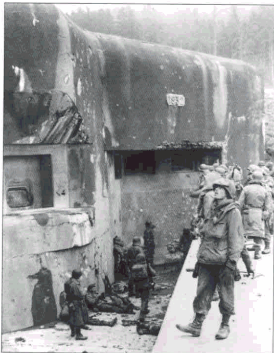
American soldiers at the gros ouvrage of Hochwald in the Vosges mountains, December 1944. They are standing in front of block 13, an unusual block that combines a casemate-mounted 135mm howitzer (the left embrasure) with a standard infantry casemate block (the right embrasures). (National Archives and Records Administration)
