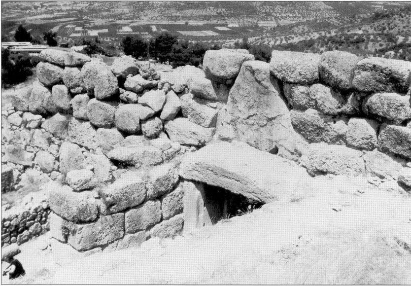
LEFT The inner façade of the Lion Gate, showing the conglomerate lintel estimated to weigh in excess of 20 tonnes. Above the lintel block, so as to reduce the load resting upon it, the wall was corbelled to leave a relieving triangle, in which is set the famous limestone relief of lions (more properly, lionesses) flanking a column, the back of which is seen here. (Author's collection)
