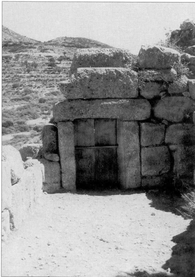
The inner façade of the North-East Postern, Mycenae's secondary gateway, which served as a ready access to the copious spring just beyond the walls to the north-east. Although much smaller, this gateway seems in style of building to be contemporary with the Lion Gate, that is, it was part of the second building phase (mid LH IIIb). (Author's collection)
