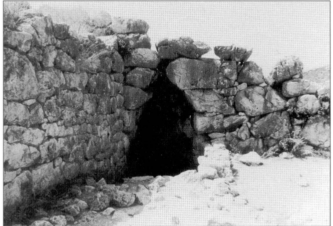
ABOVE When the inhabitants realised that Mycenae lacked an adequate supply of water to withstand a prolonged siege, they remedied the problem by extending the fortifications to the north-east, the third and final building phase of the citadel (end LH IIIb). Fresh water was then transported via gravity-fed pipes from springs in the hills to the east to a subterranean cistern. Known as the Secret Cistern, this was excavated just outside the new fortification walls, and was accessed via an elaborate descending stepped passage with a concealed entrance, seen here, just inside the curtain-wall. (Author's collection)
