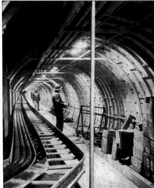
ABOVE: Work on the main tunnel of Titan I complex at Vandenberg AFB nears completion in 1960. Located 40ft. underground, the tunnel connected the launch center to the missile launch silos. (National Air and Space Museum, Smithsonian Institution)
