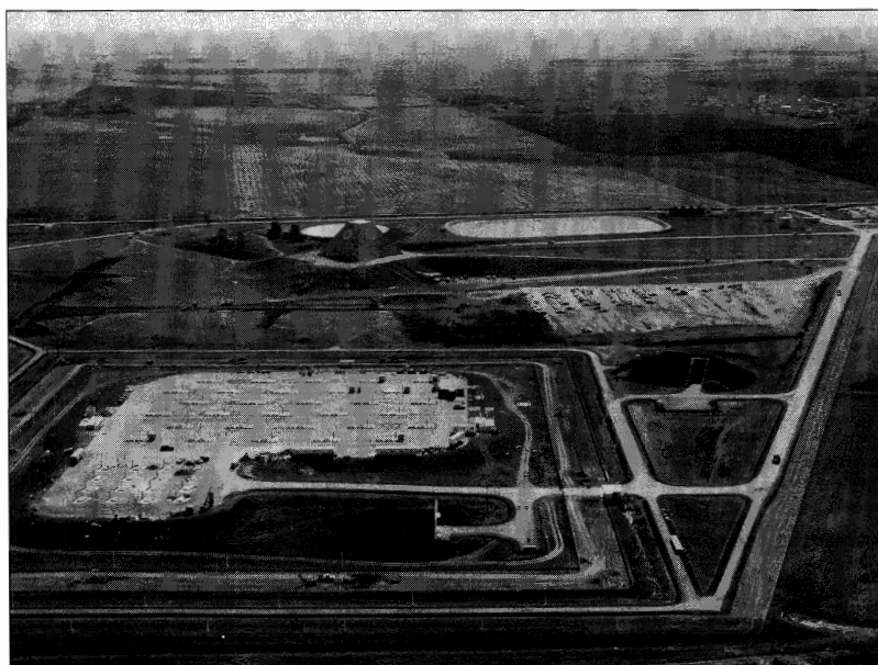
Aerial view of the main missile launch site for the Grand Forks Safeguard site. The Sprint/Spartan launch cells are located in the foreground, the pyramidal Missile Site Radar Building (MSRB) is in the upper center of the photograph. (US Army Space and Strategic Defense Command History Office, Huntsville, AL)
