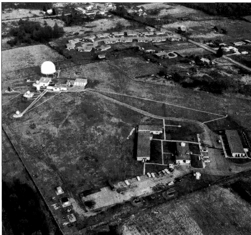
Nike-Hercules battery control site S-61 in the Seattle defense area, 1971. The administration area buildings are located to the lower right, the radars to middle left. (Courtesy Col. Milton B. Halsey, Jr.)
