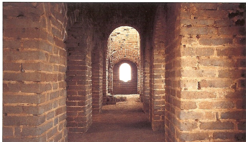
In most towers the room entered from the walkway is a gloomy cellar-like structure composed of interlocking brick arches, as in this example at Jinshanling.
