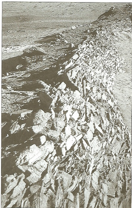
ABOVE Where there were plentiful deposits of loose stone around it was sensible to use this material for wall building. A suitable stone, simply prised from the ground, could be arranged very effectively by an experienced dry stone waller, who would use small stones to lock the larger ones together and present as smooth a face as possible to the enemy. Properly done they could be very stable structures up to 6m high. This photograph is of a Han dynasty wall in Inner Mongolia.
