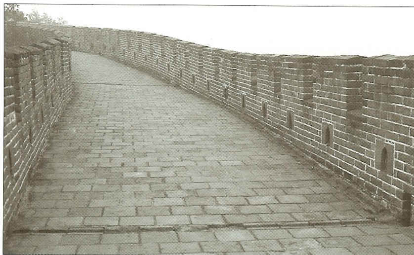
The walkways along the tops of the wall were often wide enough to allow five people to walk side by side. Where the slope is gentle the walkway slopes with it. This example is in Mutianyu, where loopholes may be also be noted.
