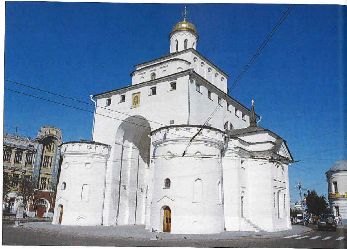
The Golden Gate in Vladimir built supposedly in the mid 12th century. It was flanked with buttresses enclosed in small circular towers and had its upper part together with the church completely rebuilt in the late 18th/early 19th centuries.
