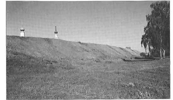
A 220m-long section of the rampart is all that remains of the fortifications of Pereyaslavl-Ryazanski, capital of the Ryazan principality from the mid 14th century. With wooden walls surmounting the rampart even the domes of the churches were not visible from beyond the fortifications.
