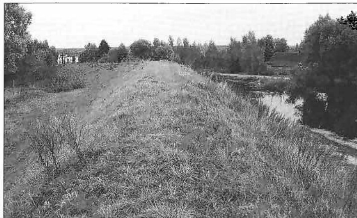
The rampart of Mstislavl. An oak intra-rampart structure has been discovered inside it. Wooden walls stood on top of the rampart, which was steeper on the exterior than on the interior. Grass, bushes, and trees on the outer side and in front of the rampart were destroyed in times of danger to prevent the enemy from hiding in them or more easily climbing the rampart.
