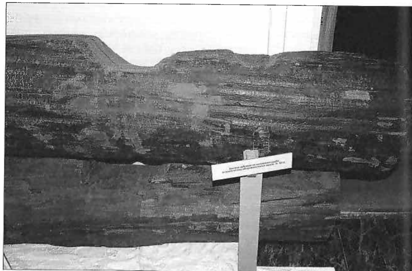
12th-century oak logs discovered in the ramparts of Vladimir. Such logs were used to build an intra-rampart structure, giving it its steepness whilst preventing the earth from sliding down. (Historical Museum in Vladimir)
