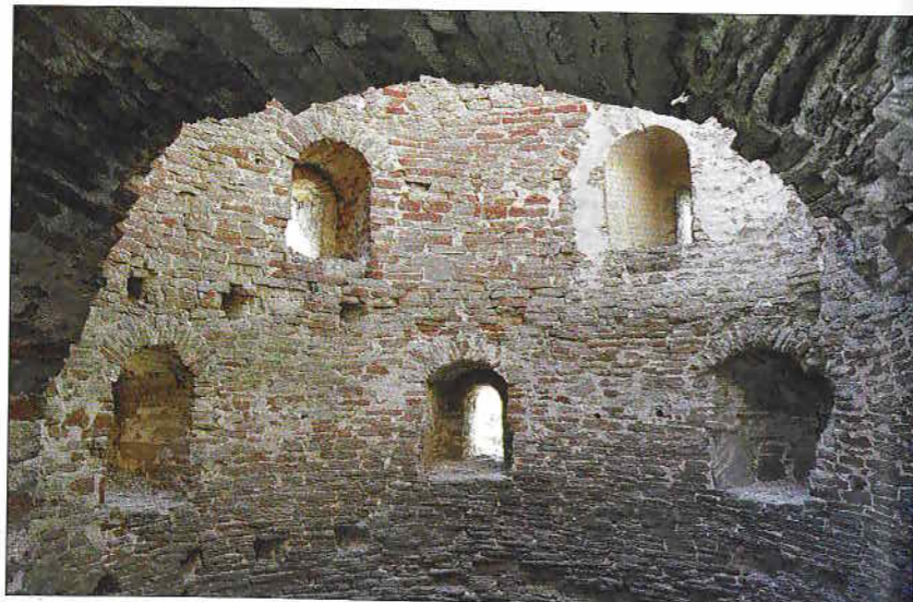
Loopholes in the Vyshka Tower. This was one of the four circular towers of Izborsk fortress, which were built in the late 14th century and modernized in the early 15th and then early 16th centuries. The loopholes are clearly arranged not one above the other but in a 'chessboard' fashion, to eliminate dead ground. On the left, between the storeys, are three square sockets left by the beams of the ceiling.
