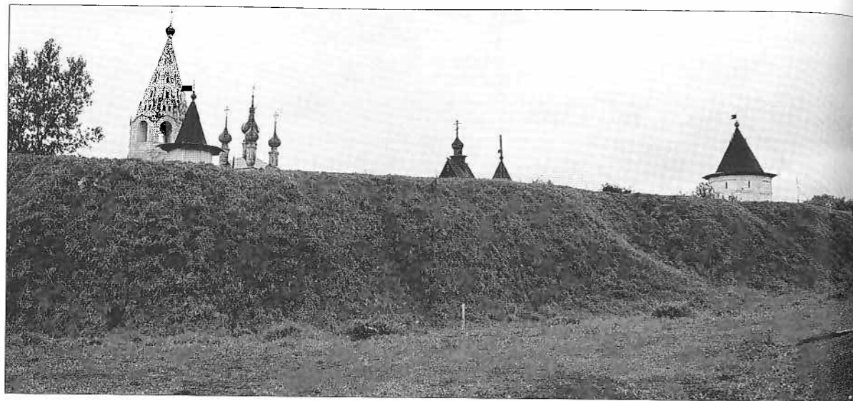
The rampart of Yuriyev-Polski, built in the 12th century. The roughly 1 km-long rampart surrounded a settlement that was almost circular in plan. As usual, the rampart was topped with wooden walls. The roofs of a later monastery are visible beyond the rampart.
