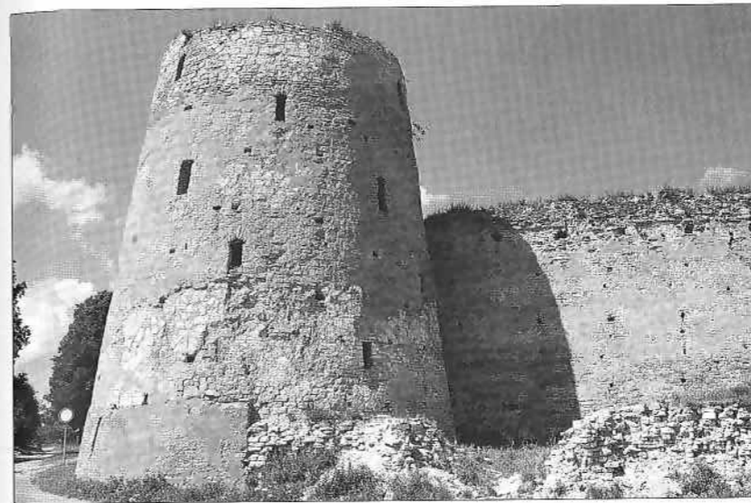
Until the very end of the 15th century towers in Russian fortresses narrowed markedly towards the top. For example, the Temnushka Tower in Izborsk fortress, seen here, has a truncated cone in shape. Visible in the foreground are the ruins of the outer wall of the Nikolski zakhab that started at this point.
