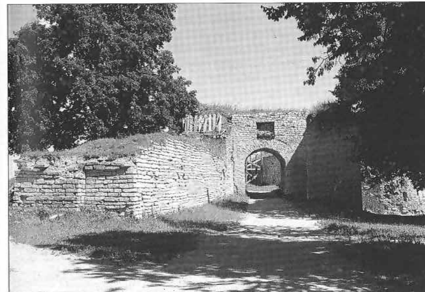
Remains of the Nikolskaya Tower, Izborsk fortress. It was raised in the 17th century at the end of the Nikolski zakhob , a long passage between the fortress walls that improved the defences of the entrance. The walls of the zakhob survive only in small sections.
