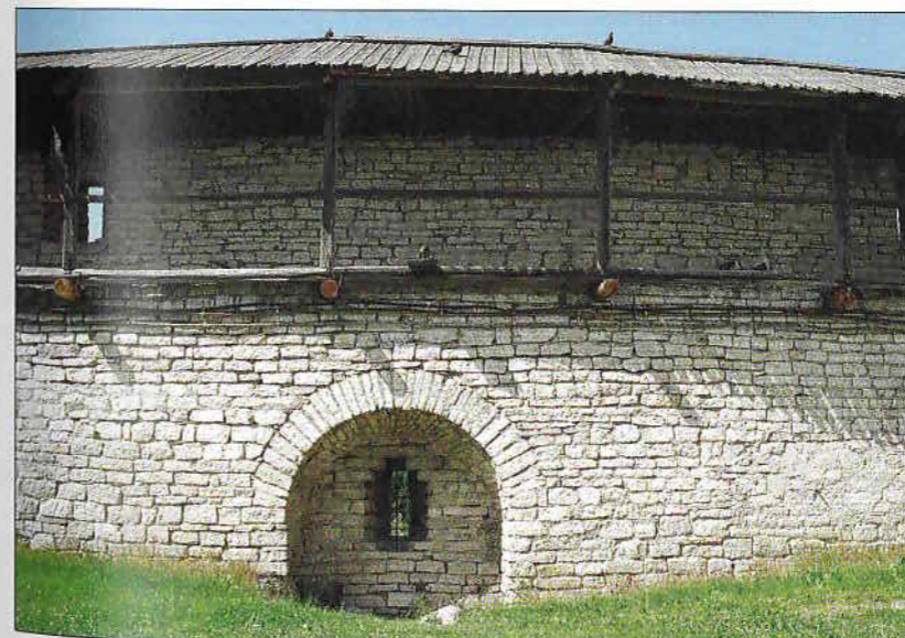
Interior view of a wall and a loophole of the boevoy hod (wall-walk) in the Pskov krom . Pskov's defensive walls lack merlons and crenellations. The parapet is solid and fire was only effected through loopholes.
