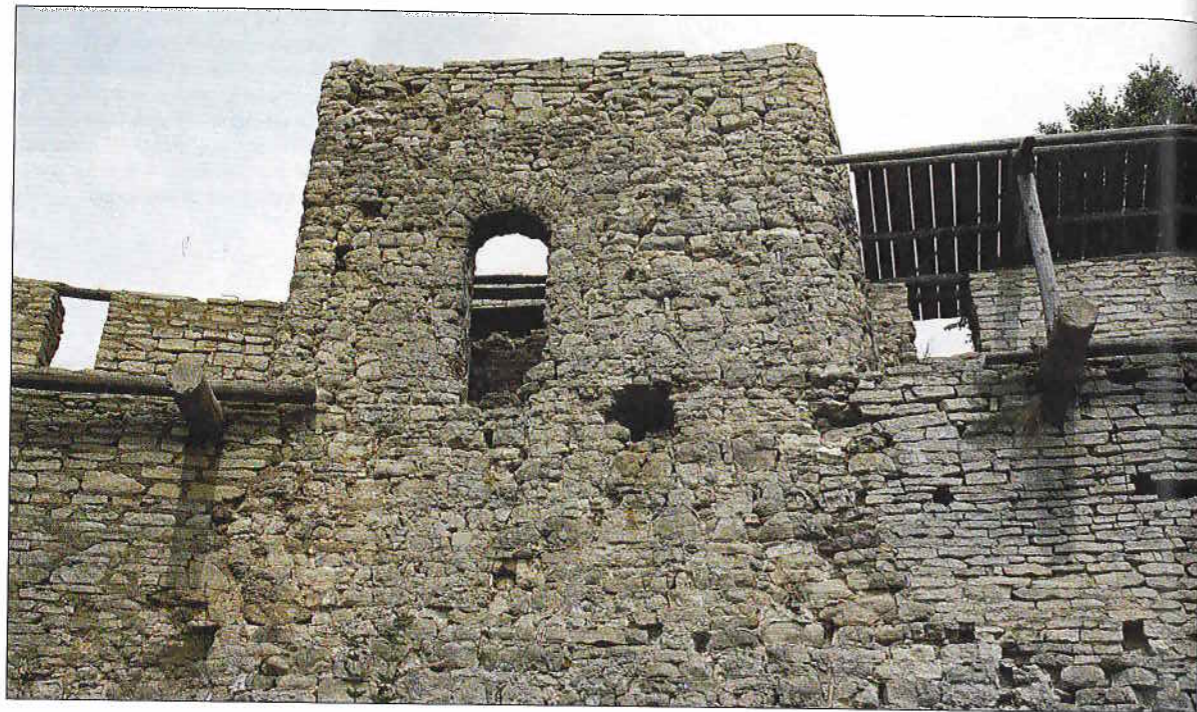
Interior view of the Malaya Tower of Porkhov fortress. The exit onto the walls here is on the rear side of the tower, on the level of the wall-walk. There would be a temporary wooden platform here, which could be easily destroyed in the event that the enemy seized the wall.
