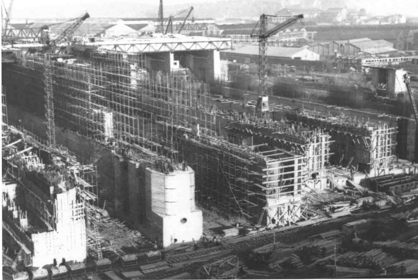
Above: U-boat pens. As well as gun emplacements, the Germans built a series of massive structures to house their submarines at various places along the Atlantic Wall. The photograph shows building in progress at the French port of Bordeaux in 1942. Bundesarchiv
