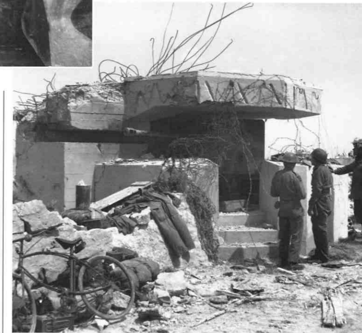
Below: Bombing and accurate naval gun fire did untold damage to the supposedly impregnable Atlantic Wall, as can be seen here on this casemate containing a 5cm KWK L/42 anti-tank gun, being inspected by Allied troops. IWM — B5252
