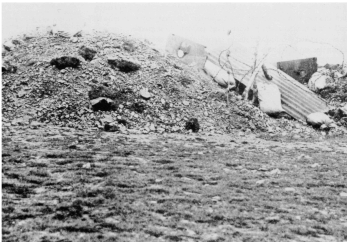
A typical German trench. Two steel sniper plates are visible (upper right), but both are for effect only. The actual sniper's loophole is inside the piece of bent iron on the left of the photo. (Author's collection)
