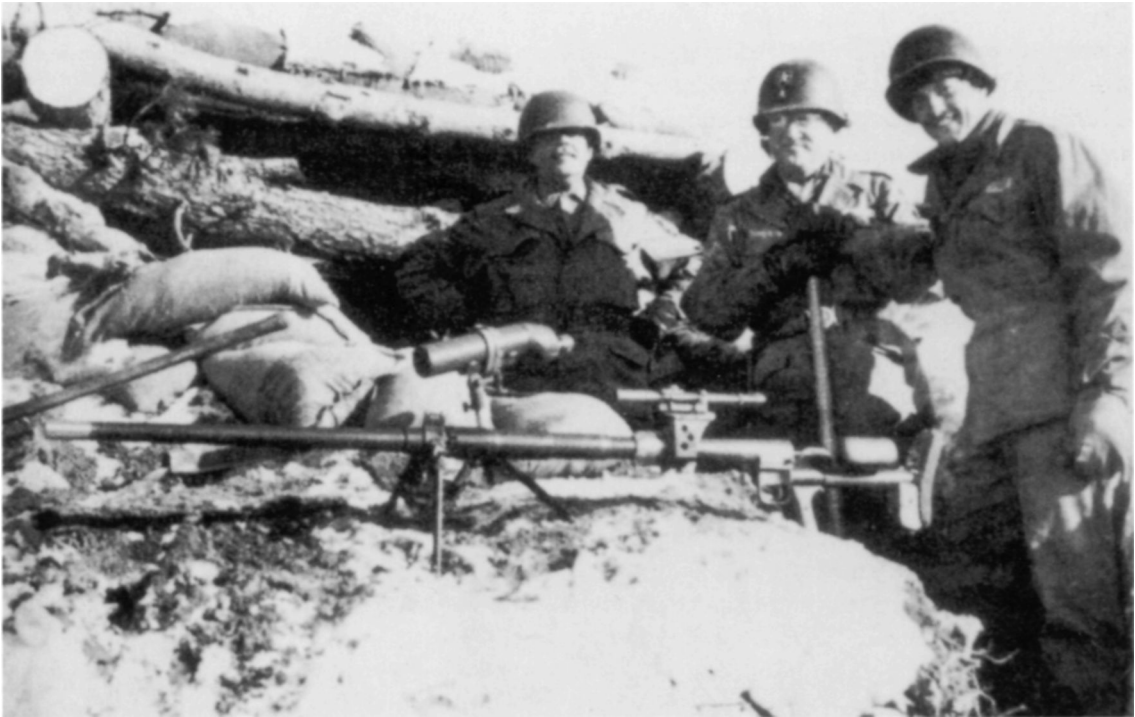
American officers pose in Korea with a Soviet PTRD anti-tank rifle that has had its barrel replaced with that of a .50 calibre Browning. In view of the potential range of this rifle the little 2.5x scope seems rather inadequate. (US Army Historical Institute)
