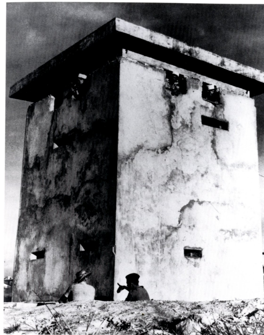
Mon Cai, January 18, 1951: legionnaires peer from a watchtower in the Red River Delta defenses. This example seems to have concrete skinning over old brick, and predates the massive “De Lattre Line” construction effort later that year, which was prompted as much by fears of a Communist Chinese conventional invasion as by hopes of stopping Viet Minh infiltration. A 235-mile arc of 1,200 prefabricated concrete blockhouses, proof against 155mm shells, were built in groups of three to six around the outer perimeter of the Delta; an inner belt 35 miles long protected the Haiphong base areas. This program required some 2,950 metric tons of concrete to be delivered every single day for a year. It completely absorbed French engineer assets and resources and much of the local economy, and was a huge financial drain. (Képi Blanc)
