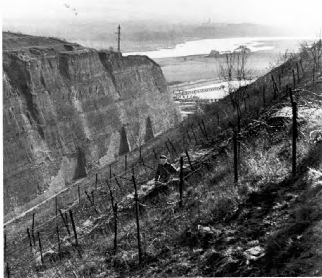
RIGHT From Eben-Emael above the Albert Canal, the Maas is overlooked to the south-east. (B751/96/27A)
