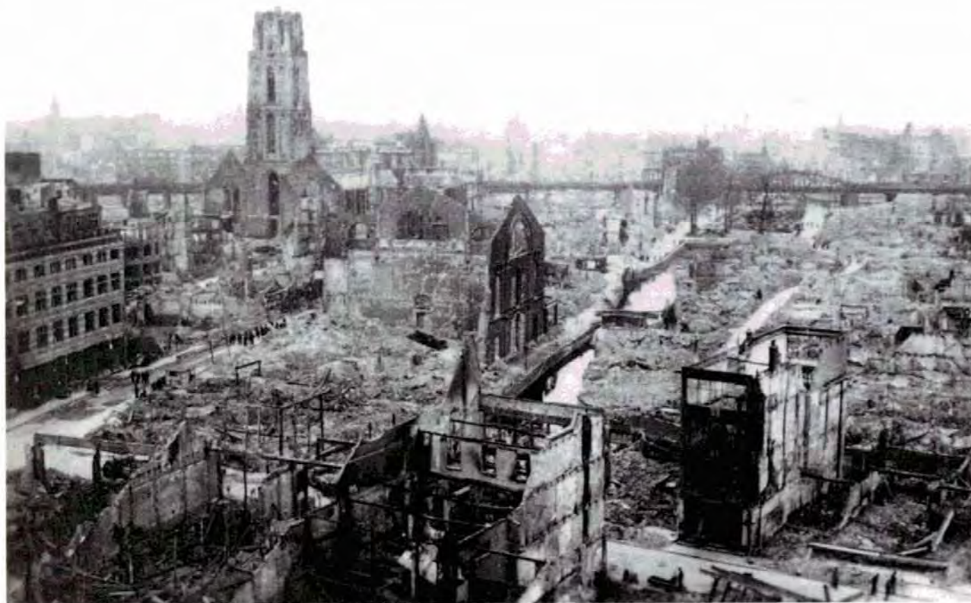
ABOVE The bombed heart of Rotterdam. The Laurenskerk is on the left and the bridge to the right carries the railway. (Photo A. C. Duijvestijn)
