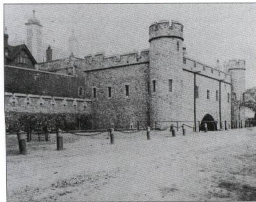
ABOVE A photograph of St Thomas's Tower taken shortly before June 1862 when part of the south-east turret collapsed. Note the tarpaulin in front of Traitors' Gate, intended to provide privacy for the soldiers of the garrison who used the water-filled basin below the building as a sort of large bathing pool! (G. Parnell)
