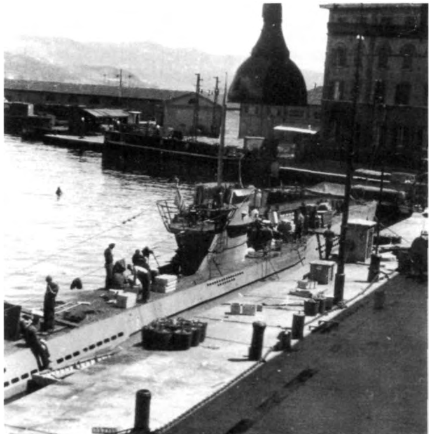
Prior to the construction of the massive concrete U-boat pens, boats were required to moor in the open. Loading large quantities of stores into a U-boat through narrow hatches was a laborious and time-consuming business during which the boat was extremely vulnerable to attack.
