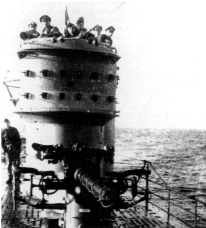
FuMB antennas, as shown here, were fitted directly to the face of the conning tower casing. The major problem with this type of antenna is that it could only cover the area in front of the boat, so that the boat would have to cruise round in a circle to obtain 360-degree cover
