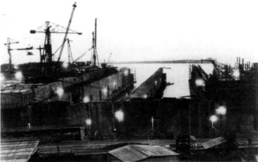
The Brest bunker gradually takes shape. Powerful arc lights installed throughout the site enable work to continue virtually around the clock. Attempts to disrupt construction of the U-boat bunkers in France through Allied bombing raids were relatively ineffective.
