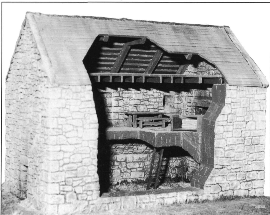
This model gives a good idea of the construction and strength of the bastle or ‘bastell howse’ which once predominated in the Border country. Most bastles have no more than three small windows, these invariably being set high up in the wall. The wooden ladder giving access to the small, stout external door would be pulled up by the inhabitants in times of trouble. Bastles were virtually fire proof and as a further precaution stone roofing tiles were secured with sheep bones. (Border History Museum, Hexham)
