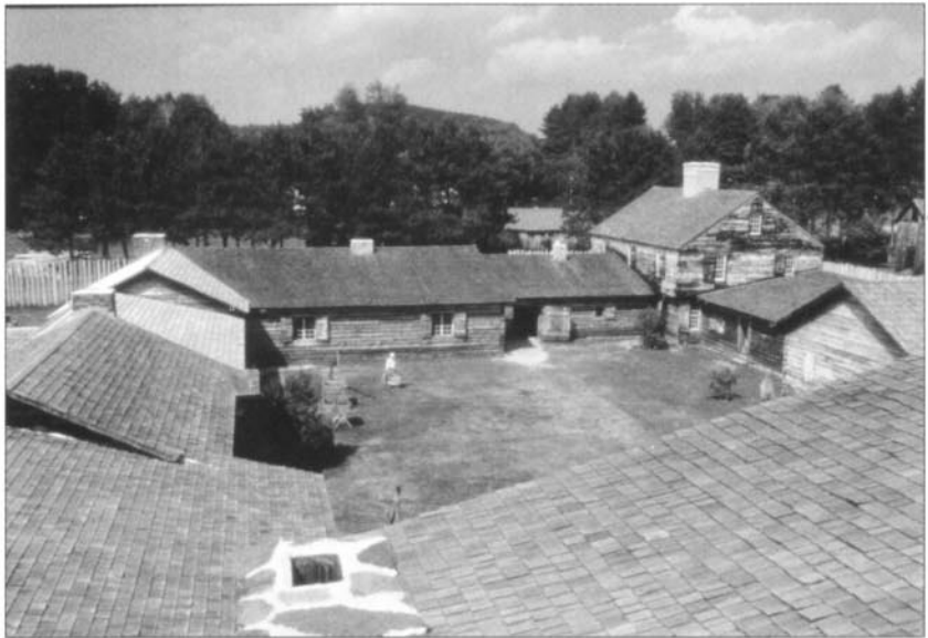
View of the interior of Fort No. 4 as it might have appeared in the 1740s–50s. As can be seen, the houses of the settlement's inhabitants were clustered together to form a fort, the outside walls being sturdy and pierced with loopholes. Small pieces of ordnance could be mounted on the second stories of the corner buildings. This type of fort-settlement was not exceptional and could also be found on the frontiers of Pennsylvania and Virginia. (Photo: RC)
